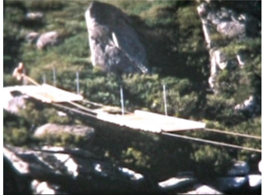
**Photo No. 29 Pulling assembled wooden deck sections across the Snowy (John Turner)**
