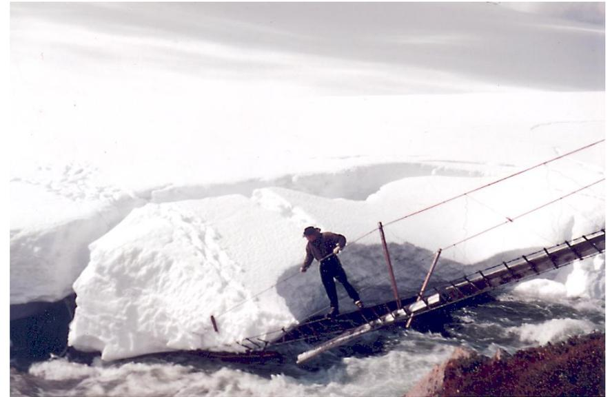
**Photo No. 32** Flood Damage to Illawong's First Bridge (Toni Smith 1958)
